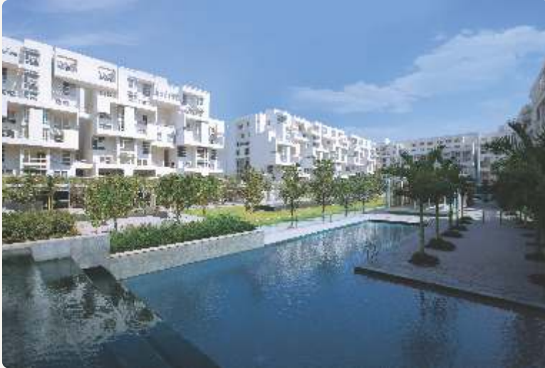
Rohan Mithila, Opp. Airport, Pune.
