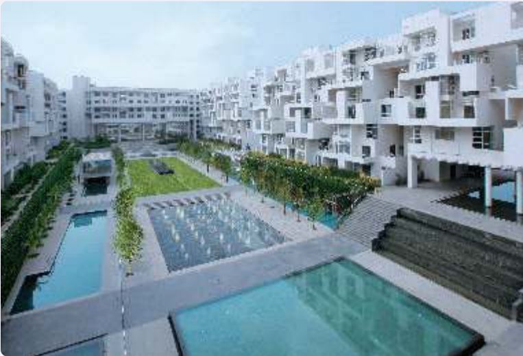
Rohan Mithila, Opp. Airport, Pune.
